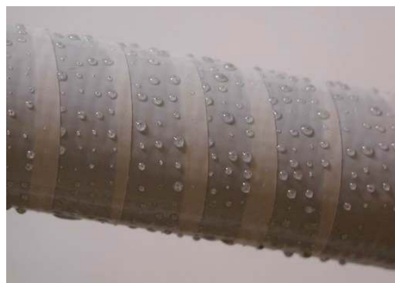
Fig. 14. Excess resin after wrapping
